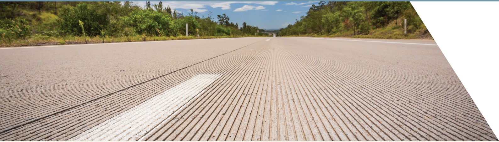
Hunter Expressway Concrete Pavement, showing a Diamond Grooving technique applied.
